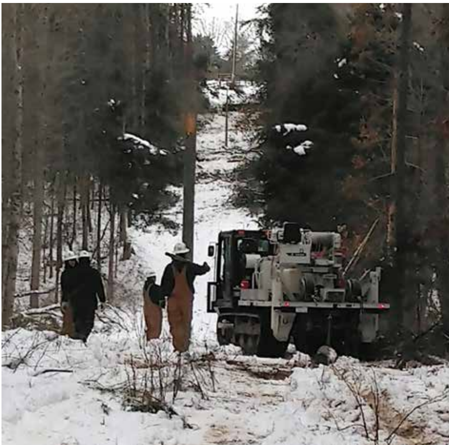
MARK CRAMER/LEAD LINEMAN
